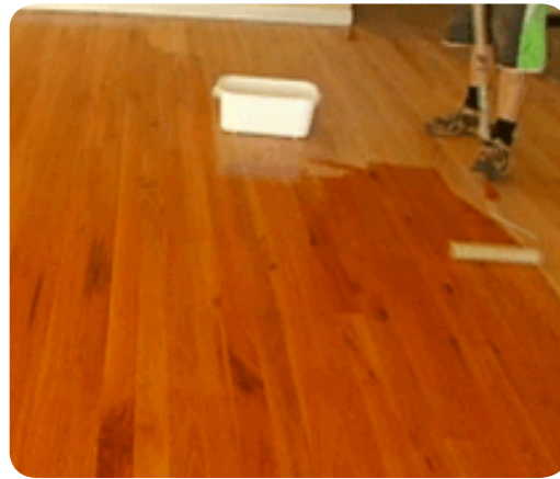
Figure 8.10: Application of the initial coat.
