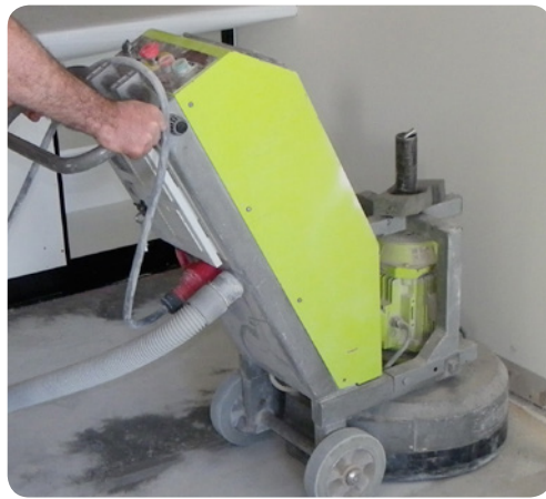
Figure 5.3: A slab being ground flat, which also removes contaminants.
