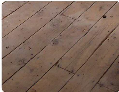
Figure 4.13: Before laying over existing floors, the moisture content and structural integrity needs to be assessed.
