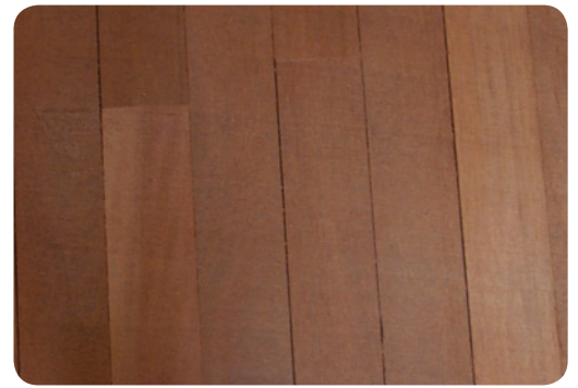
Figure G2: Wide gaps due to high moisture contents at the time of machining.
