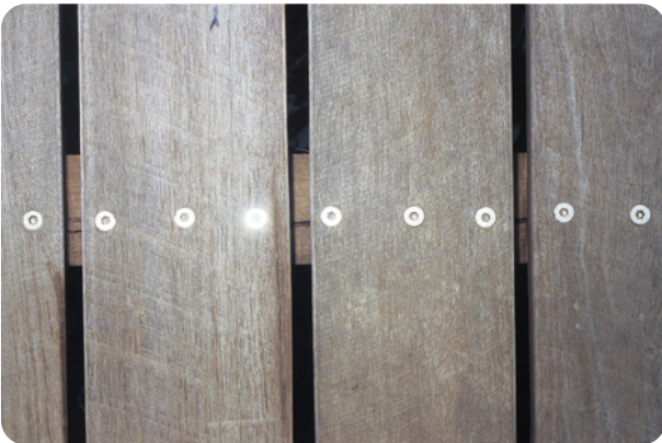
Deck screws have been staggered to prevent splitting of joists.
