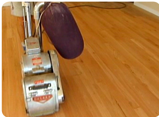
Figure 8.6: The finish sand.
