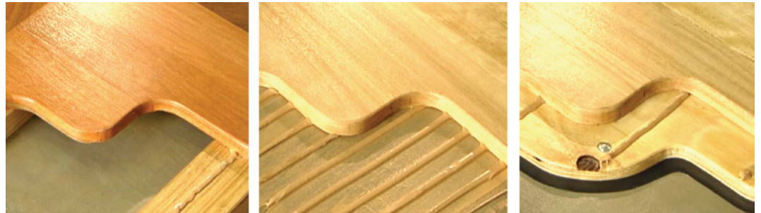
Figure 4.17: Methods to lay timber floors over concrete slabs include battens, direct adhesive fix and over plywood. Direct adhesive fix should be undertaken by professional floor installers.
