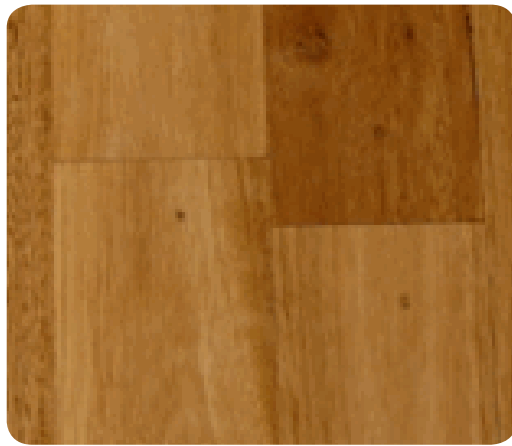
Figure 9.3: Boards ends should be spaced out and preferably 450 mm or more apart.
