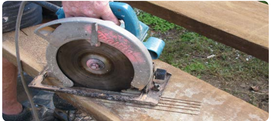
Figure 5.10: Housing strings.
