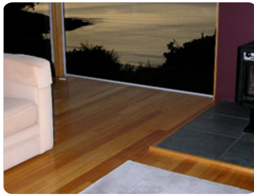
Figure 3.14: Window tinting or low emissivity glass should be considered with floor to ceiling windows to reduce shrinkage effects from direct sun.
