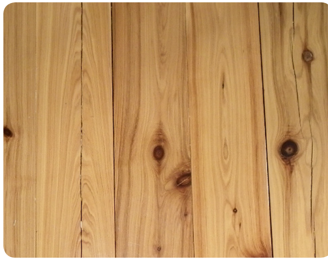
Figure 3.21: Edge bonding can result in wide irregularly spaced gaps at board edges and split boards within the floor.
