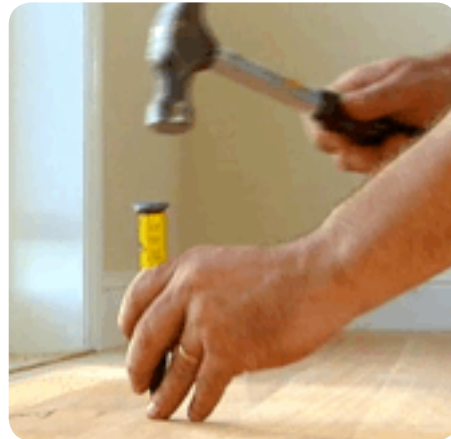
Figure 8.2: Nails are to be punched and holes filled.
