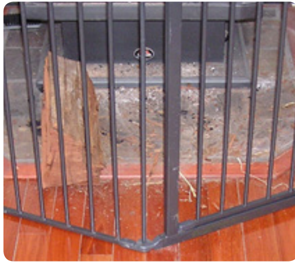
Figure 3.11: Intense heating sources can cause localised shrinkage.
