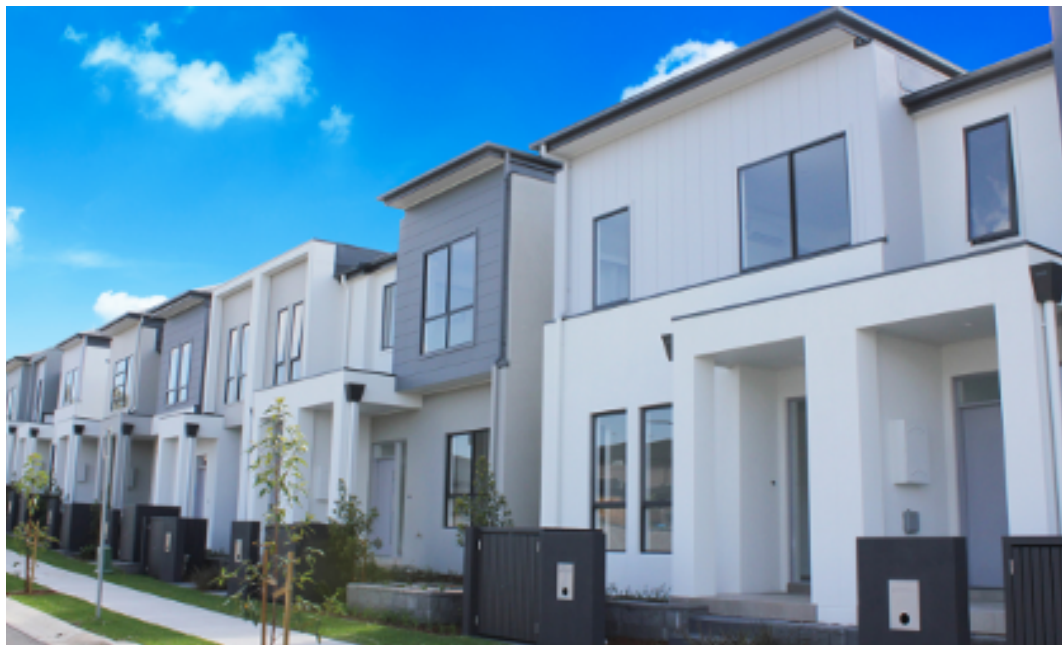
Figure 10: Two-storey Class 2 or 3 building with direct access to an open space or road. (Image: Weathertex)
