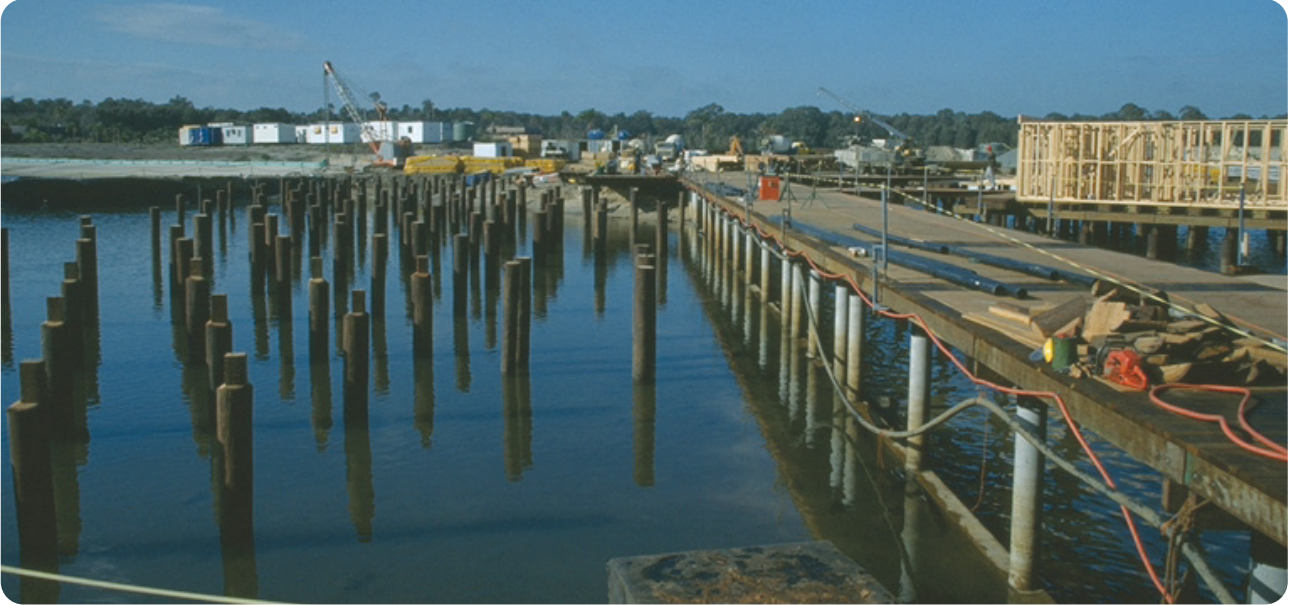
Double treated marine piles at Couran Cove, Queensland.
