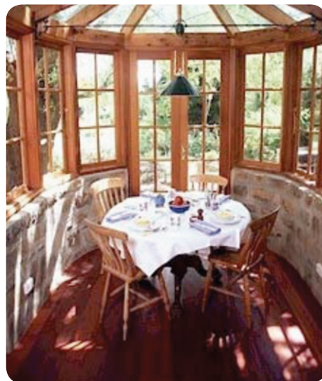
Figure E2: Sydney Blue Gum floor with underfloor hydronic heating.
