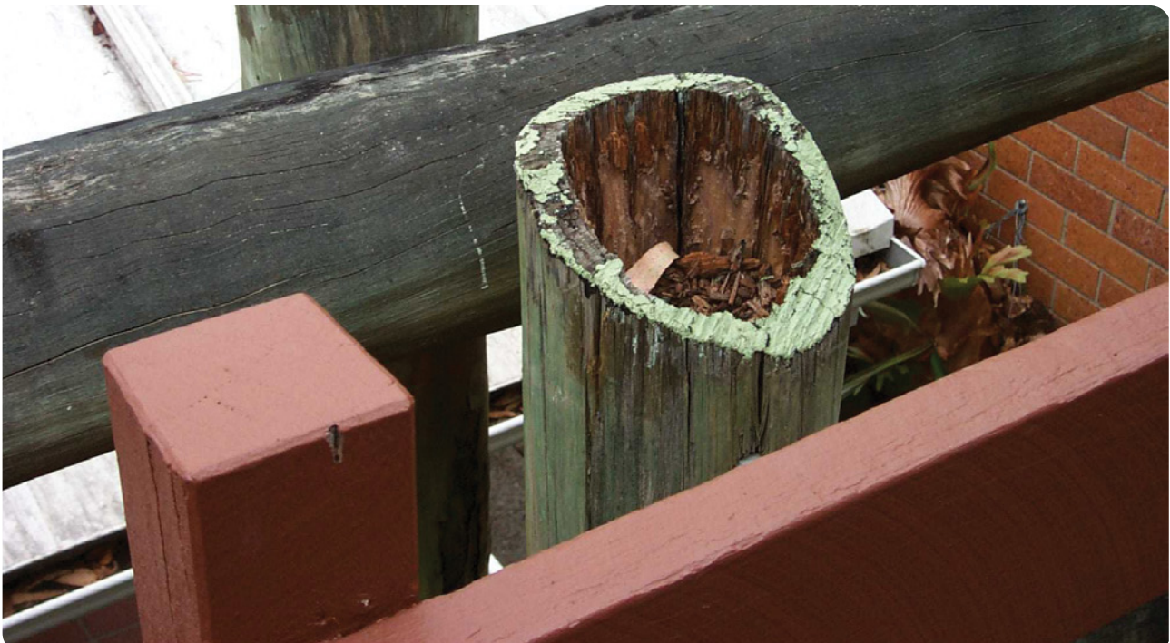
CCA treated sapwood outperforming durability class 2 heartwood.
