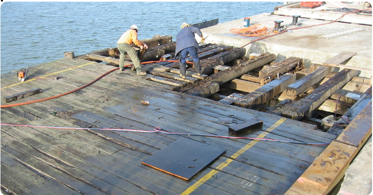
Wharf timbers to be recycled and re-used after about 60 years in-service.
