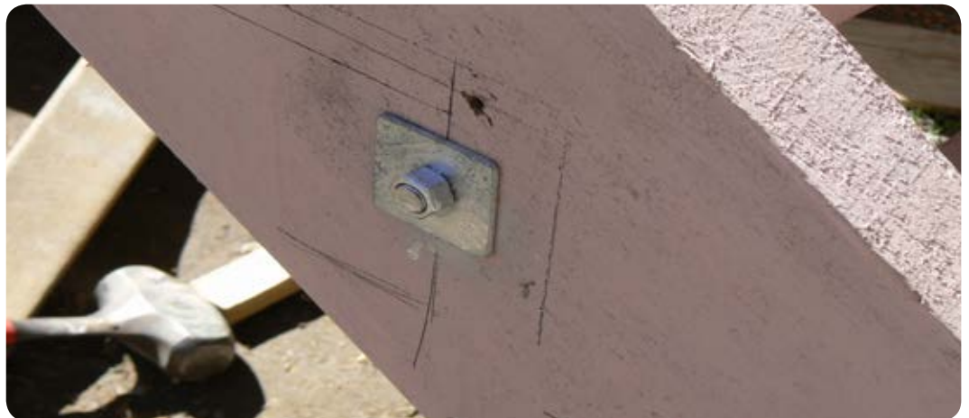
Figure 5.15: Position of step bolt.
