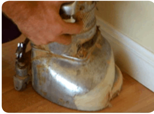
Figure 8.5: Edge sanding requires a smooth action to blend into the floor.
