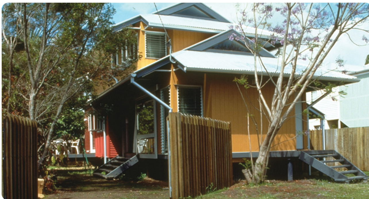
Large overhangs provide good protection.
