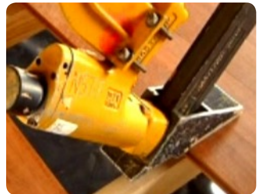
Figure 4.12: Secret fixing is recommended for boards up to 85 mm in cover width.
