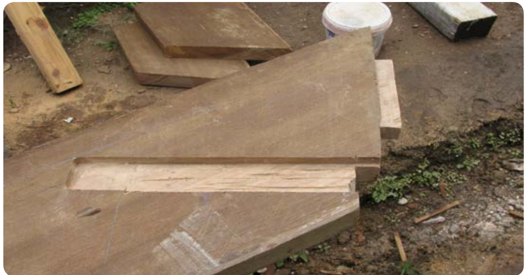
Figure 5.12: Supporting stringers.
