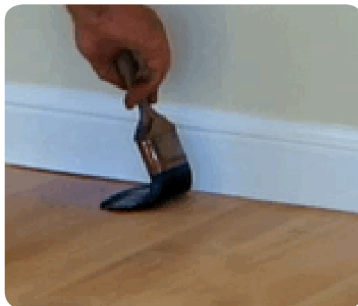
Figure 8.9: Cutting in the finish around perimeter walls.
