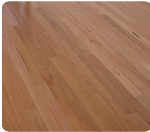
Figure 9.2: A select grade Blackbutt floor where the backsawn gum vein toward the top right exceeds grade limits but is acceptable within the floor.
