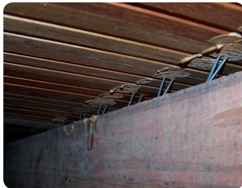
Figure 4.9: Buckling of 80-mm-wide Spotted Gum boards secretly fixed to pine joists in a humid locality.
