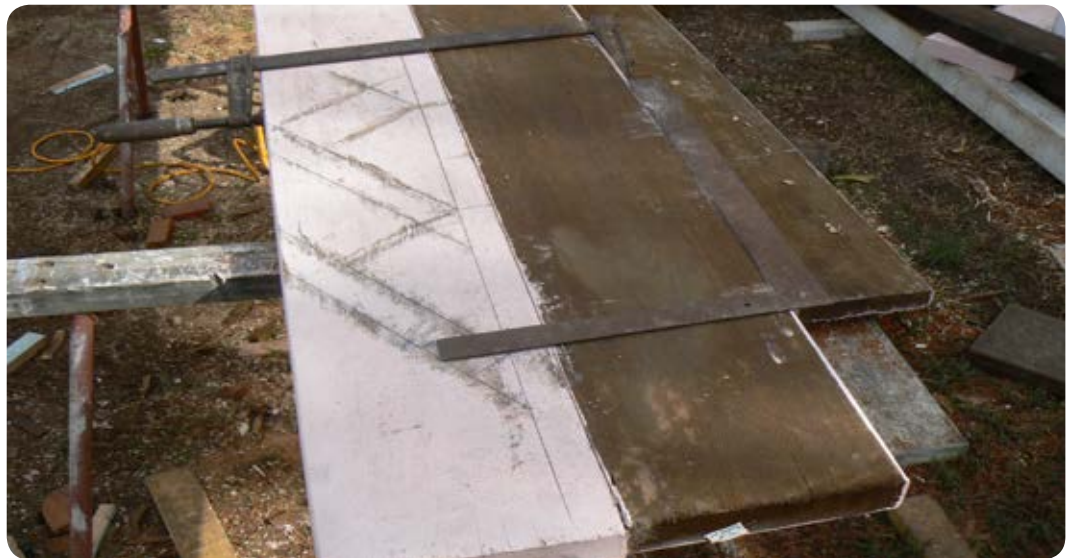
Figure 5.7: Marking out left string.
