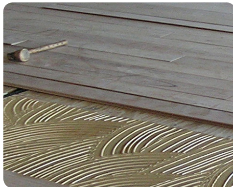
Figure 4.20: Adhesive spread prior to fixing.
