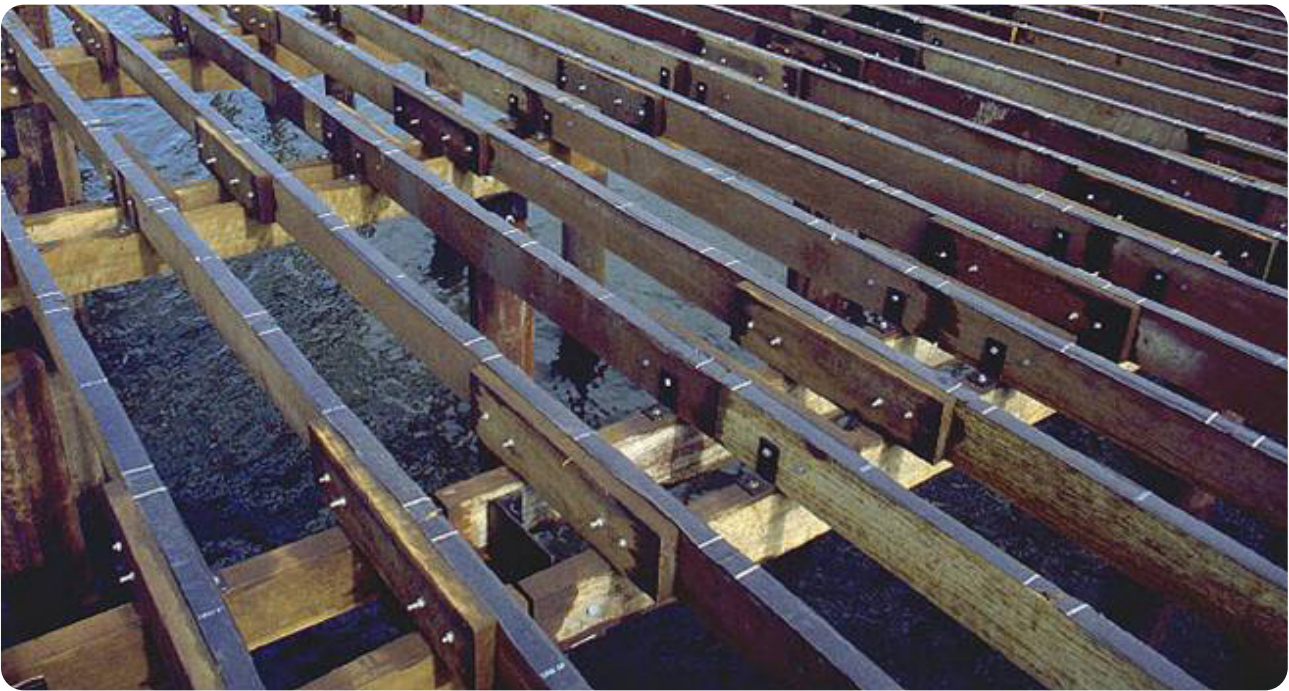
Bituminous DPC fixed to top of deck joists.
