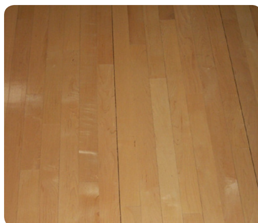
Figure 4.2: Small regular gaps can be used to provide the additional expansion allowance needed, particularly for wide floors or in moist climates. These often close during humid periods.
