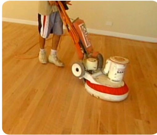
Figure 8.8: Buffing the floor.
