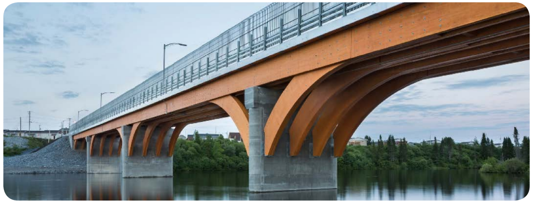
Figure 1.6: Mistissini Bridge, Canada using a CLT road platform. Photograph: Nordic Structures
