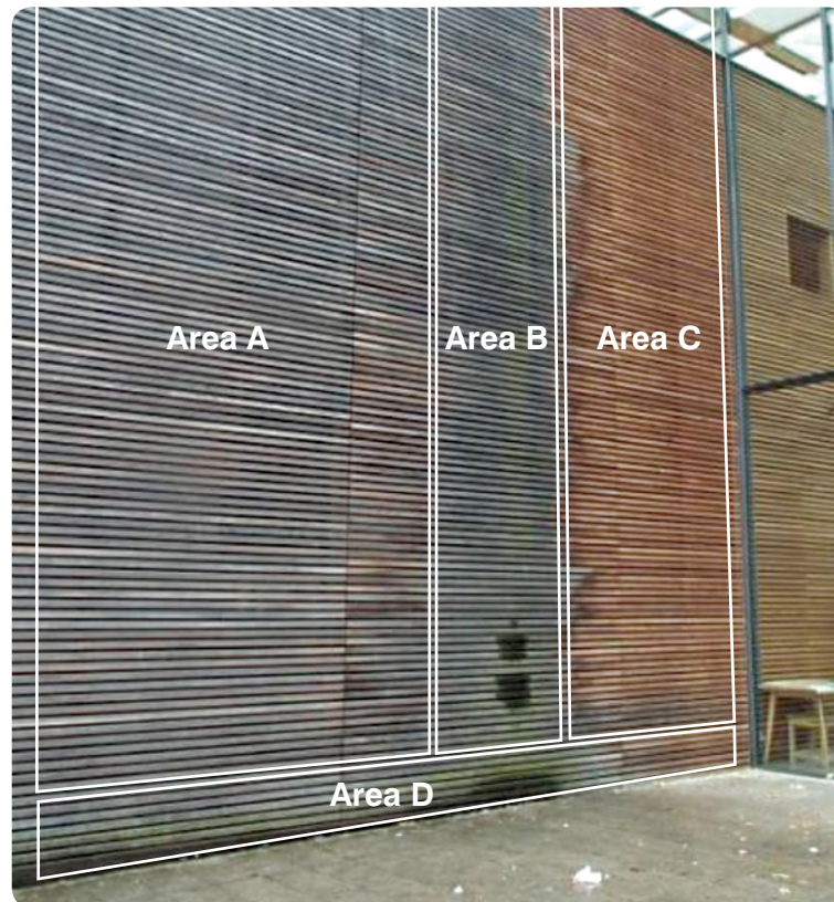
Figure 10: Differential weathering across a façade.
