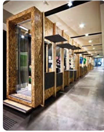
Matt Gibson Architecture and Design: The Coop - structure and cladding constructed from LVL Beams and OSB Panelling.
