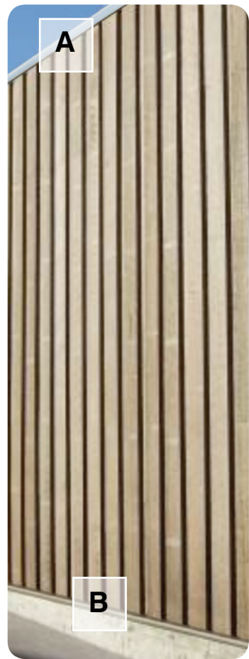
Figure 15: Detailing to avoid standing water.
