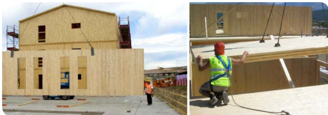
Figure 5.2: Slings and brackets used to support CLT panels during lifting.
