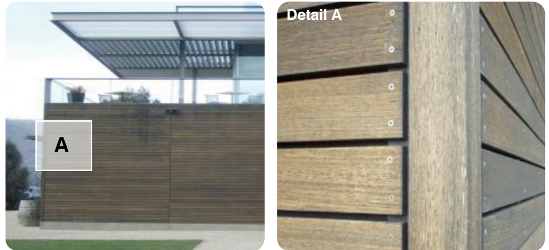
Figure 23: Visually significant fasteners, seasoned horizontal cladding.
