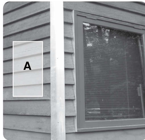
Figure 21: Detailing green timber weatherboards to allow movement.
