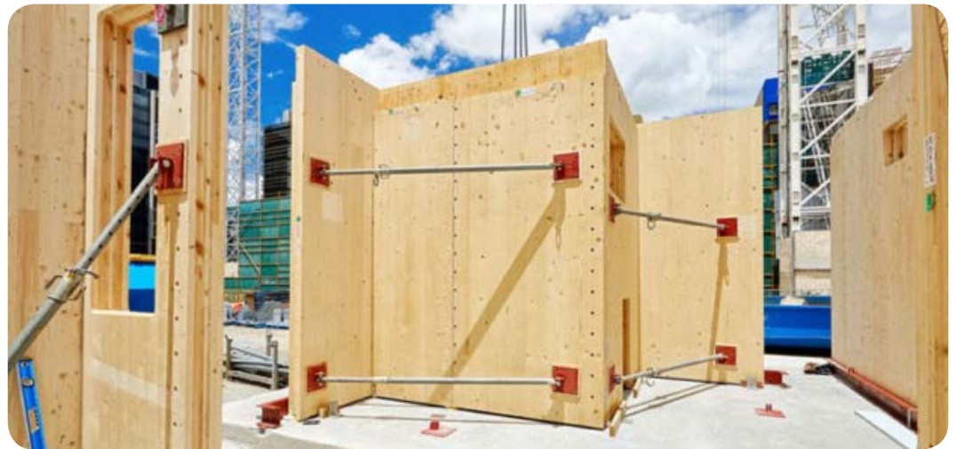
Figure 4.1: Site assembled CLT core. Photograph: Lendlease
