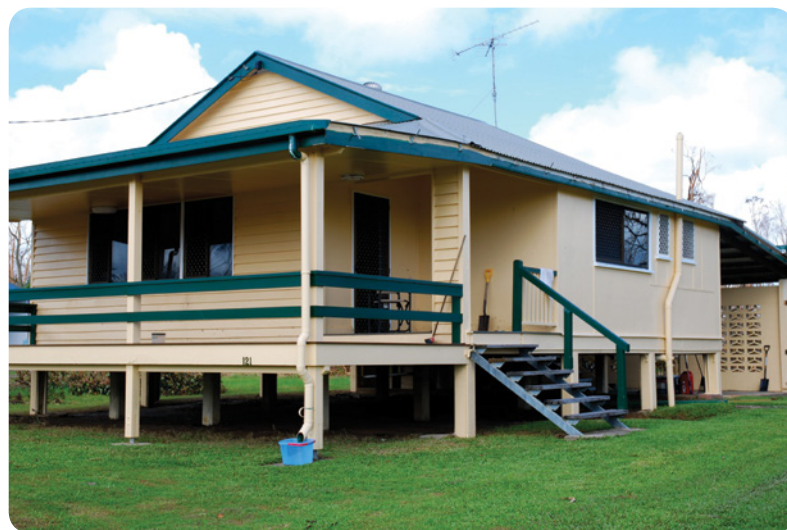
Elevated houses suffered little storm surge damage. (Image: Cyclone Testing Station, James Cook University, Townsville)
