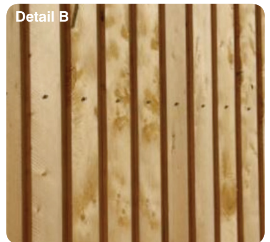
Figure 22: Visually significant fasteners; vertical green timber cladding.
