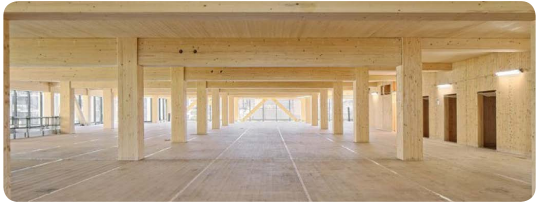
Figure 1.3: CLT used as a floor and walls inside office building, K5 Brisbane. Photograph: Lendlease
