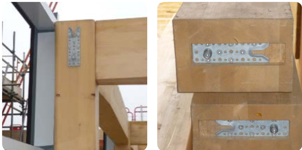
Figure 5.5: Specialist Timber Connector. Photograph: TDA
