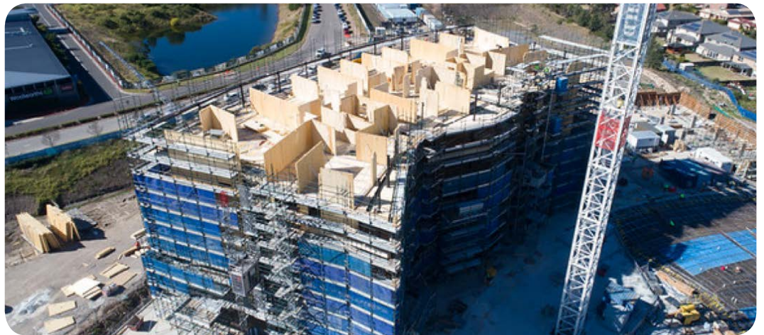
Figure 1.4: CLT used for apartment construction, AVEO Norwest. Photograph: Strongbuild
