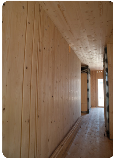
Left: Figure 7.3: Interior view of Forté prior to internal linings being affixed. Steel elements projecting into corridor are pre-fabricated bathroom pods. Photograph : Lend Lease
