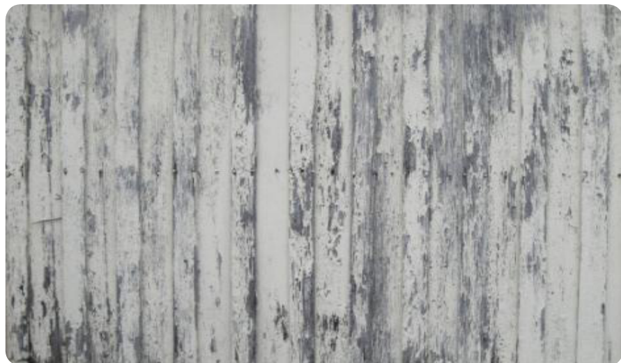
Figure 19: Poorly maintained film-forming finish.
