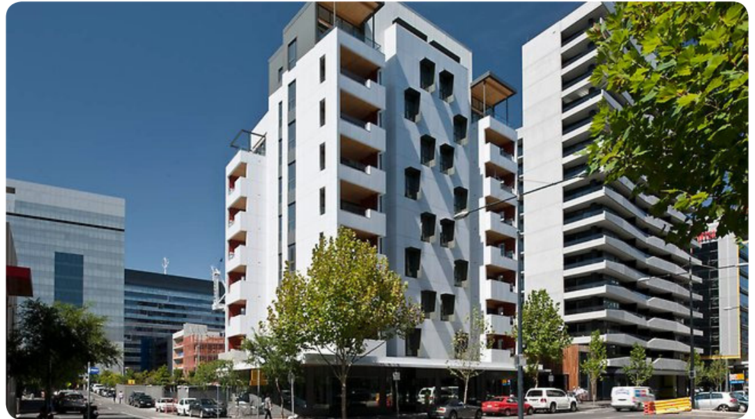
Figure 7.1: Completed Forté apartments. Photograph: Lend Lease
