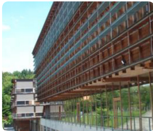
Figure 11: Sheltered bare timber.
