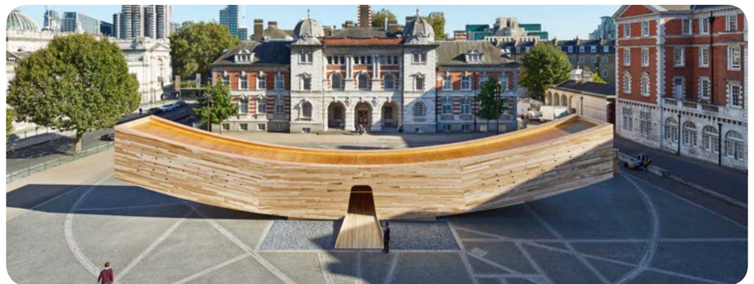
Figure 2.1: London Smile made from American tulipwood hardwood CLT
