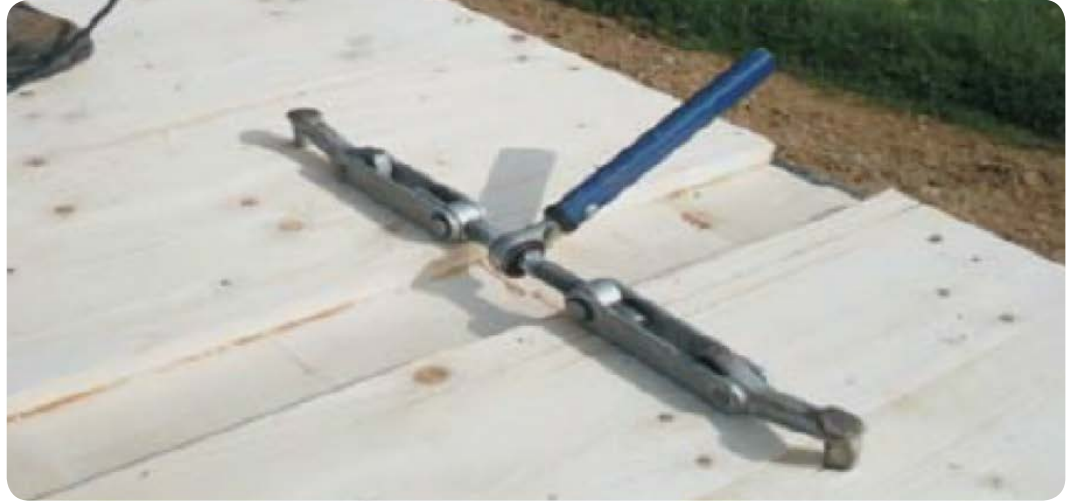
Figure 5.6: Special clamp used to align CLT floors. Photograph: WoodSolutions
