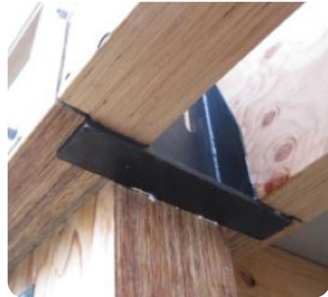
(b) Steel corbel protected with intumescent paint.
