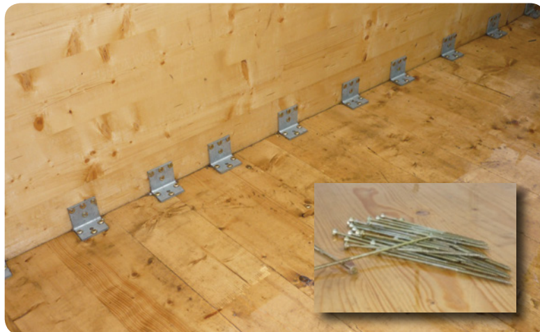
Figure 5.4: Wall to floor connection. Photograph: TDA
