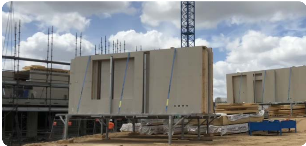
Figure 5.1: Trailers used to store panels before installation on site. Photograph: TDA
