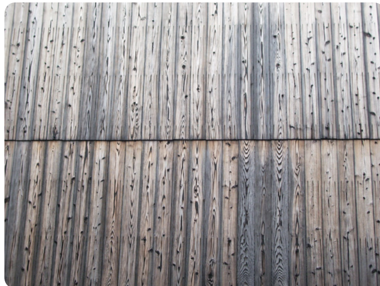
Figure 1: Bare timber used externally in a temperate climate.
