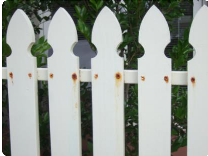
Figure 20: Rapid corrosion of poorly specified fasteners.
