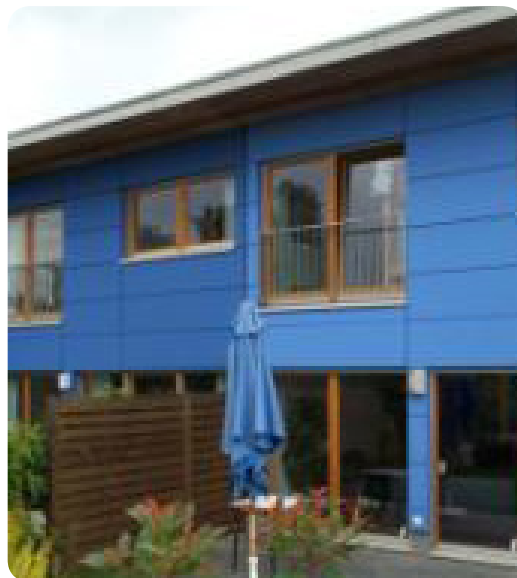
Figure 7: Painted plywood cladding, varnished timber joinery.
