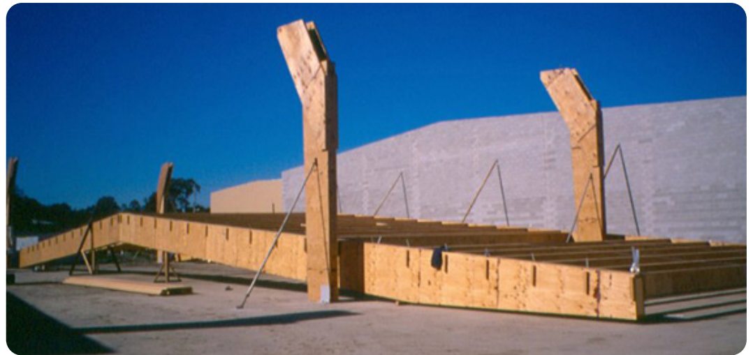
Figure 3: Timber portal roof structure constructed on the ground. Image: Timberbuilt
