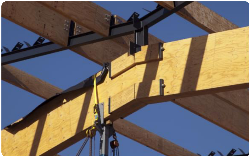
Figure 4: Quick connect moment connector in Netball Central 3 (Image: Geoff Ambler; Ethan Rohloff).
