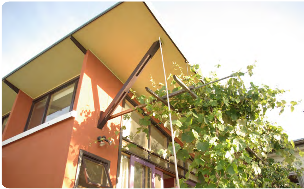
Figure 10: Blocking western summer sun. Trellises with climbing plants can be used to shield western façades. (Photo: Gregory Nolan)
