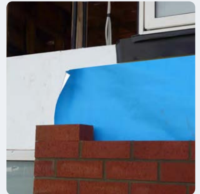
Extruded polystyrene over-cladding a timber-framed wall before external cladding is fixed.
