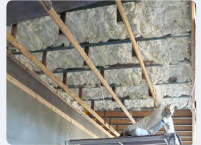
Sprayed-in-place wall insulation
