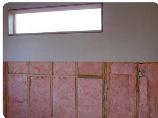
Figure 38: Correctly installed wall batts insulation. Photo: Mark Dewsbury
