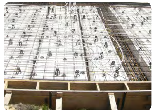
Figure 37: Underslab waffle-pods. Underslab insulation is suitable for cooler climates. Photo: Mark Dewsbury
