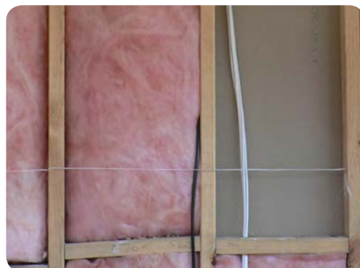
Figure 40: Batt insulation removed for installation of services. Photo: Mark Dewsbury
