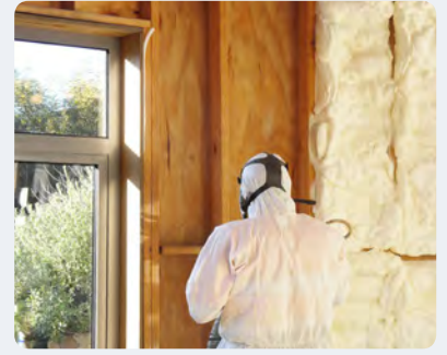
Sprayed-in-place wall insulation
