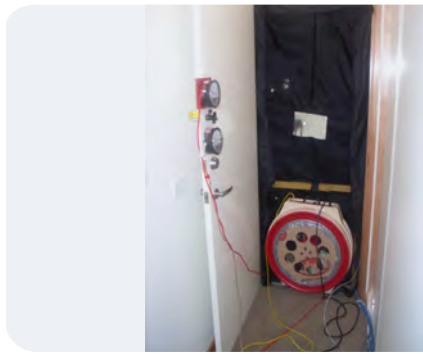
Figure 28: Blower door testing. A fan temporarily sealed in an external door allows for airtightness to be measured. Photo: Mark Dewsbury
