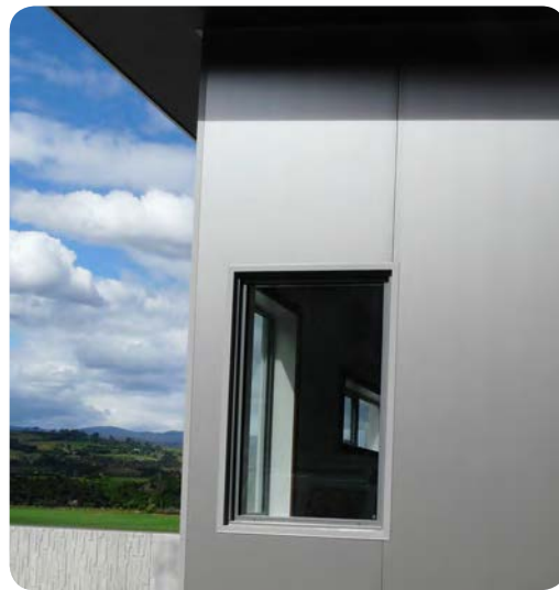
Figure 53: Rigid insulations as external cladding. Solid insulated panel with sheet-metal faces and polystyrene core. Photo: Mark Dewsbury
