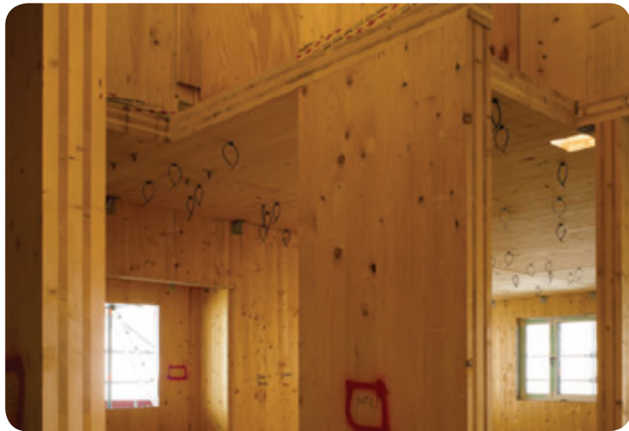
Figure 1: Cross-Laminated Timber construction.
