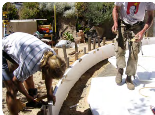
Figure 36: Board under slab and slab edge insulation. Slab edge insulation is suitable for most climates. Photo: Mark Dewsbury
