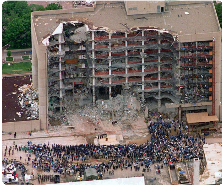
Figure 3.6: Oklahoma City's Murrah Building after the bomb attack.
