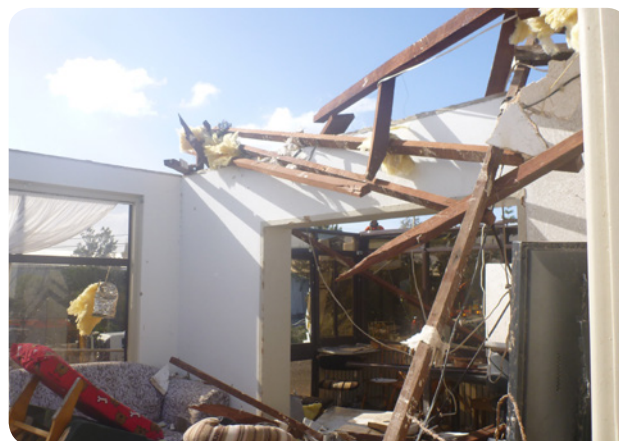
(b) Roof structure to wall connection
