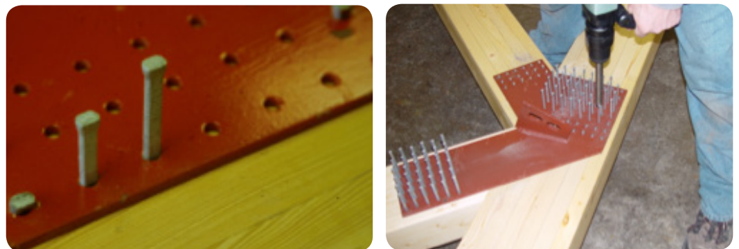
Figure 1.1: Timber rivet connections. Source: Buchanan, A., Timber design guide New Zealand Timber Industry Federation Inc. Wellington, New Zealand, 2007.
