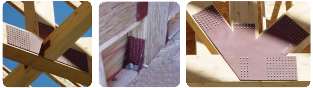
Figure 1.3: Sample applications of timber rivet connections. (Image credit: Specialized Timber Fasteners Ltd, Canada)
