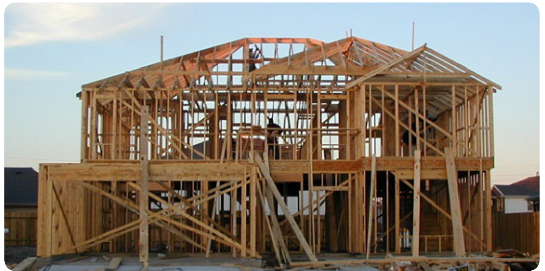
Figure 6.1: Typical timber-framed domestic construction.
