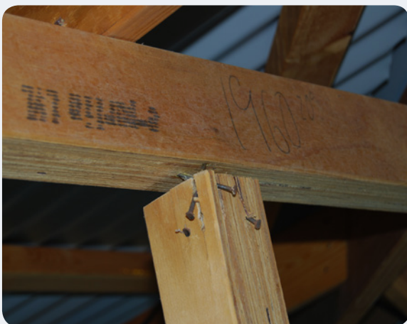
(c) Underpurlin-to-strut connection
