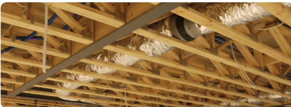
Figure 2.6: Hybrid floor system with parallel chord trusses supported from a steel I-beam.
