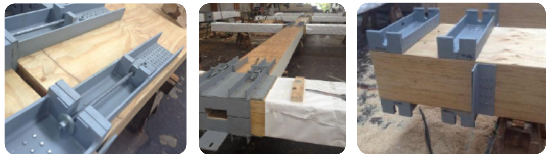
Figure 1.5: Riveted connections of the Trimble building in Christchurch, New Zealand. (Image credit: McIntosh Timber Laminates Ltd)
