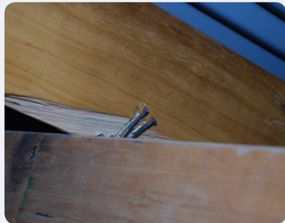
(b) Rafter-to-underpurlin connection
