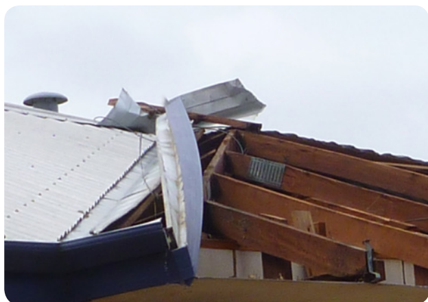
(a) Batten-to-rafter or truss connection
