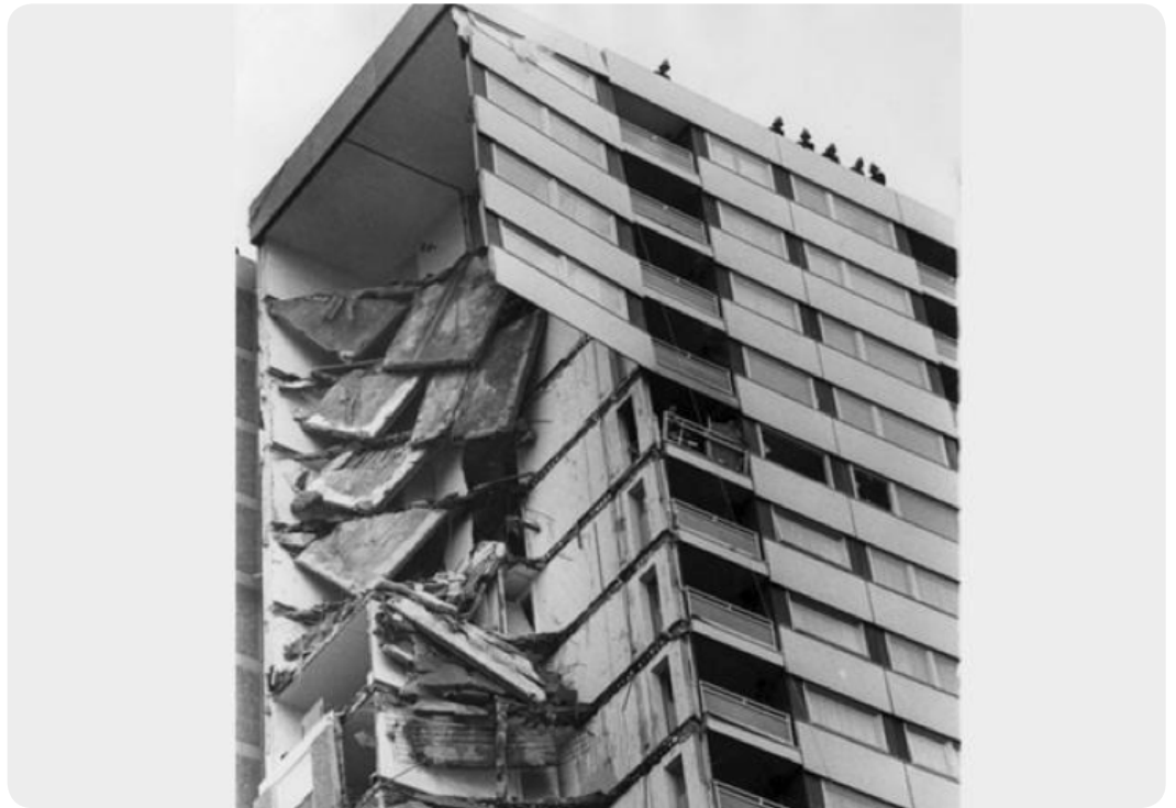
Figure 1.2: Ronan Point, UK – progressive collapse of one side of building due to gas explosion.
