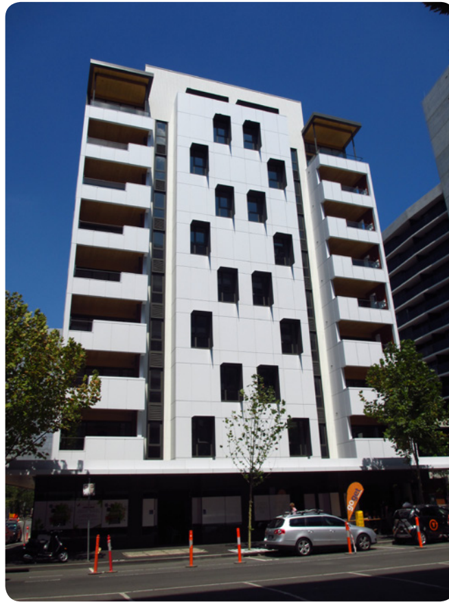
Figure 6.2: Forte, Melbourne, nine storeys of CLT on concrete podium.
