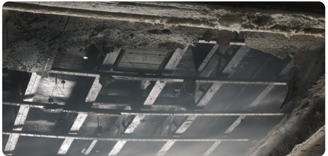
Figure E4: Fire-exposed face of lightweight loaded timber floor system about eight minutes after 90-minute fire resistance test, after suppression with a fire hose.
