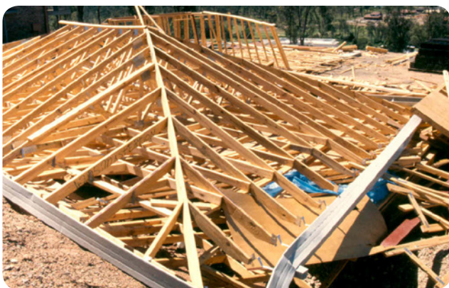
Figure 6.6: Failures of houses under construction due to inadequate temporary bracing.
