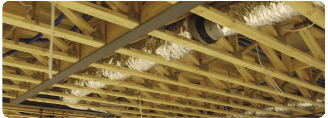
Figure 2.3: Mix of steel and timber beams in a floor.
