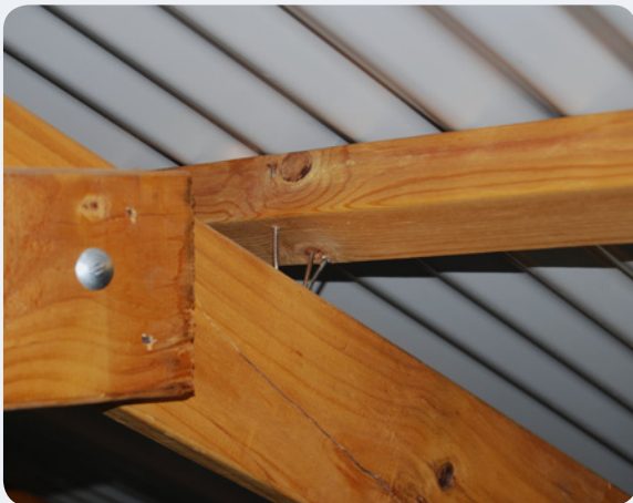
(a) Batten-to-rafter connection
