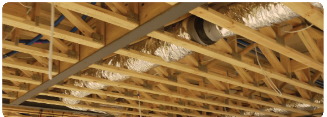
Figure 0.3: Hybrid floor system with parallel-chord trusses supported from a steel I-beam.
