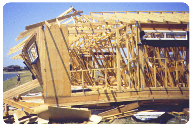
Figure 6.6: Failures of houses under construction due to inadequate temporary bracing.
