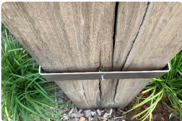
Figure 5.9: Large gaps under straps.
