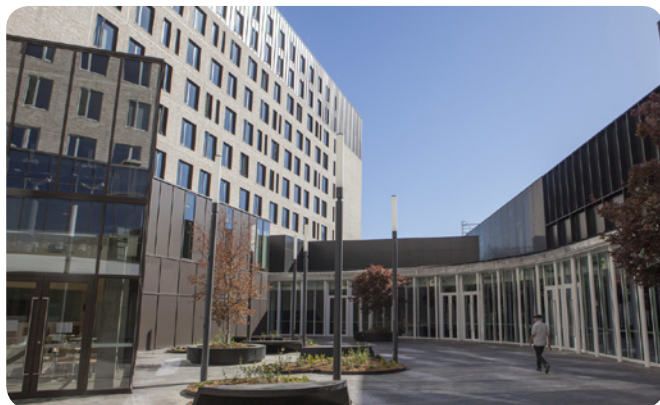
Figure 1.4 – The Kambri precinct of Australian National University (Canberra, 2019) incorporates two large mass timber construction buildings: the 450-bed student accommodation and the five-storey collaborative teaching building. Designed by BVN (architects) and constructed by Lendlease, the student accommodation was also the first building in Australia to use a new prefabricated facade system from Inclose that enabled 13-metre-long fully complete brick facade sections to be installed within 20 minutes. Images: Lendlease
