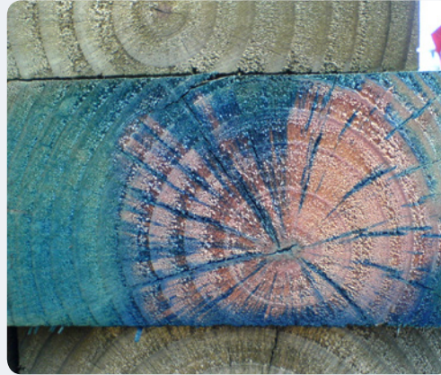
B: Softwood with insufficient incising. Good penetration of softwood treatment is dependent on incising to the correct depth. An applied stain detects the level of penetration of the preservative treatment. This pine bollard was incised to about 3 mm rather than the 10 mm required resulting in a centre vulnerable to deterioration.
