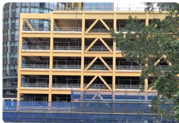
Figure 6.2: Timber Post and Beam, International House, Lend Lease (Image: TDA)
