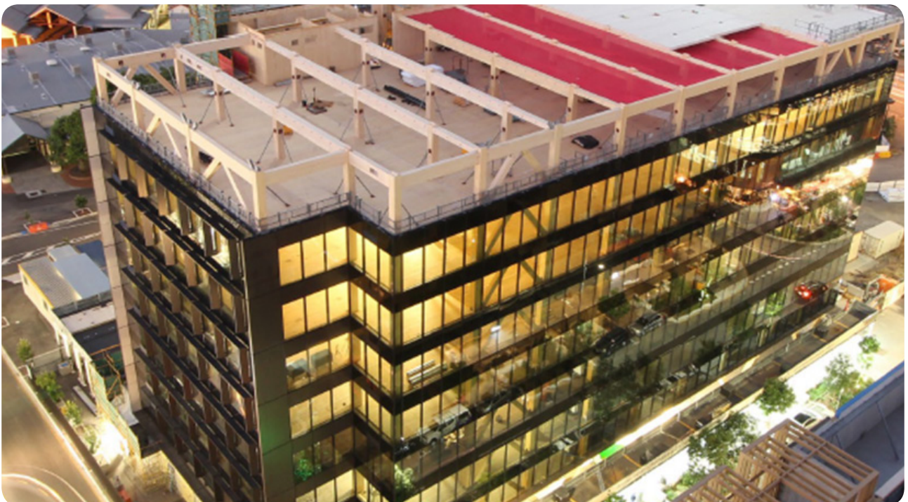
Figure 1.1: The office built by Lendlease at 25 King Street, Brisbane, embodies the advantages of timber construction for all six categories described in Figure 1.2 (Lendlease)
