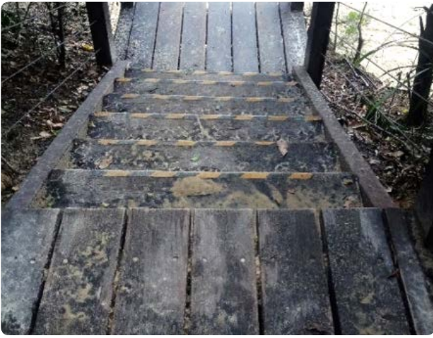
Figure 3.19: Incorrect orientation of boards at landings.
