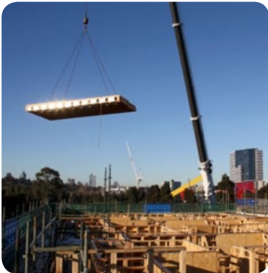
Figure 6: Prefabrication-intensive construction – panel construction.
