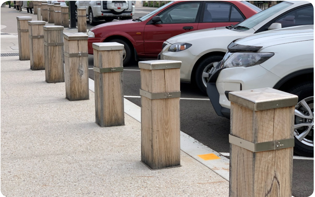
Figure 5.11: Misaligned caps.
