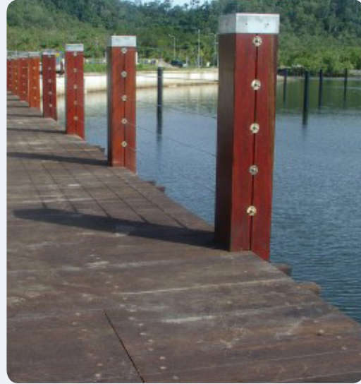
B: Balustrade – Infill cables and balustrading provide protection from falling.
