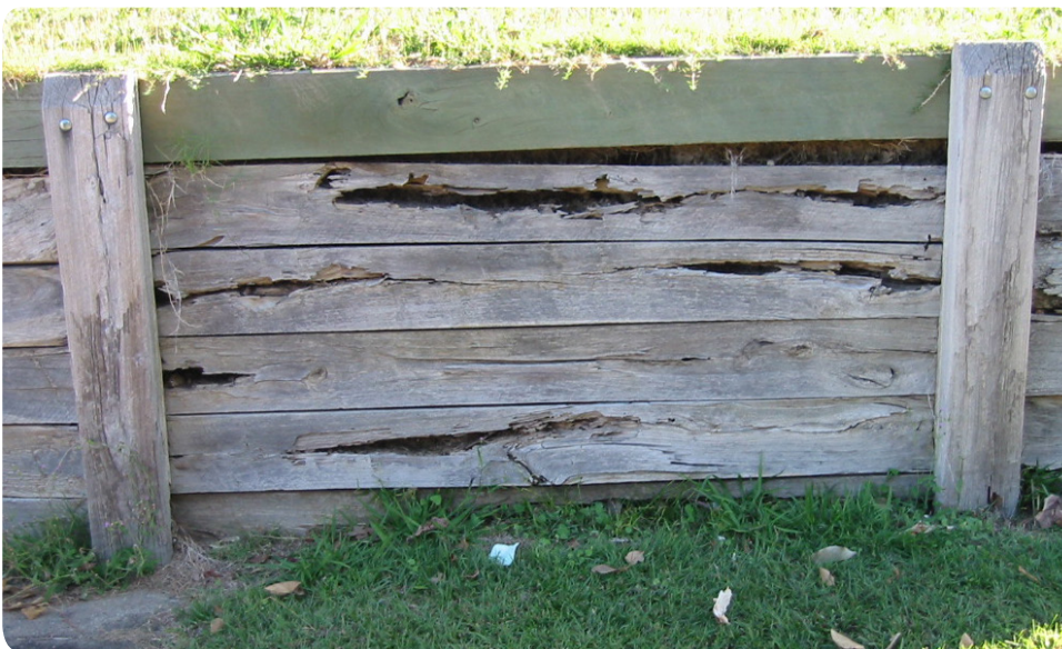
Figure 2.3: Low quality hardwood sleepers
