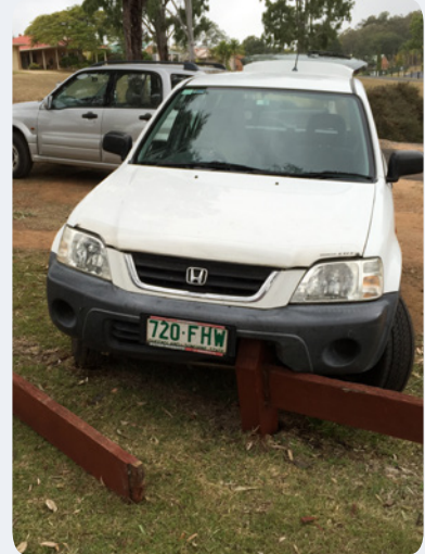
C: Hardwood barrier – The 30-year-old hardwood barrier is shown here intact despite having rendered considerable damage to the vehicle.
