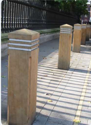
A: Mass bollards – Mass bollards from single large timber members risk environmental consequences.
