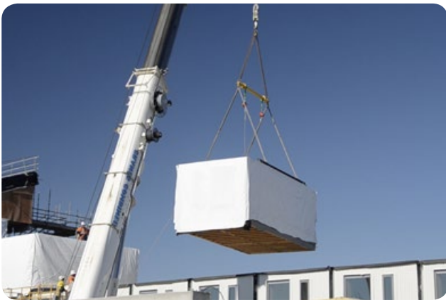
Figure 9: Prefabricated modules in installation and assembly
