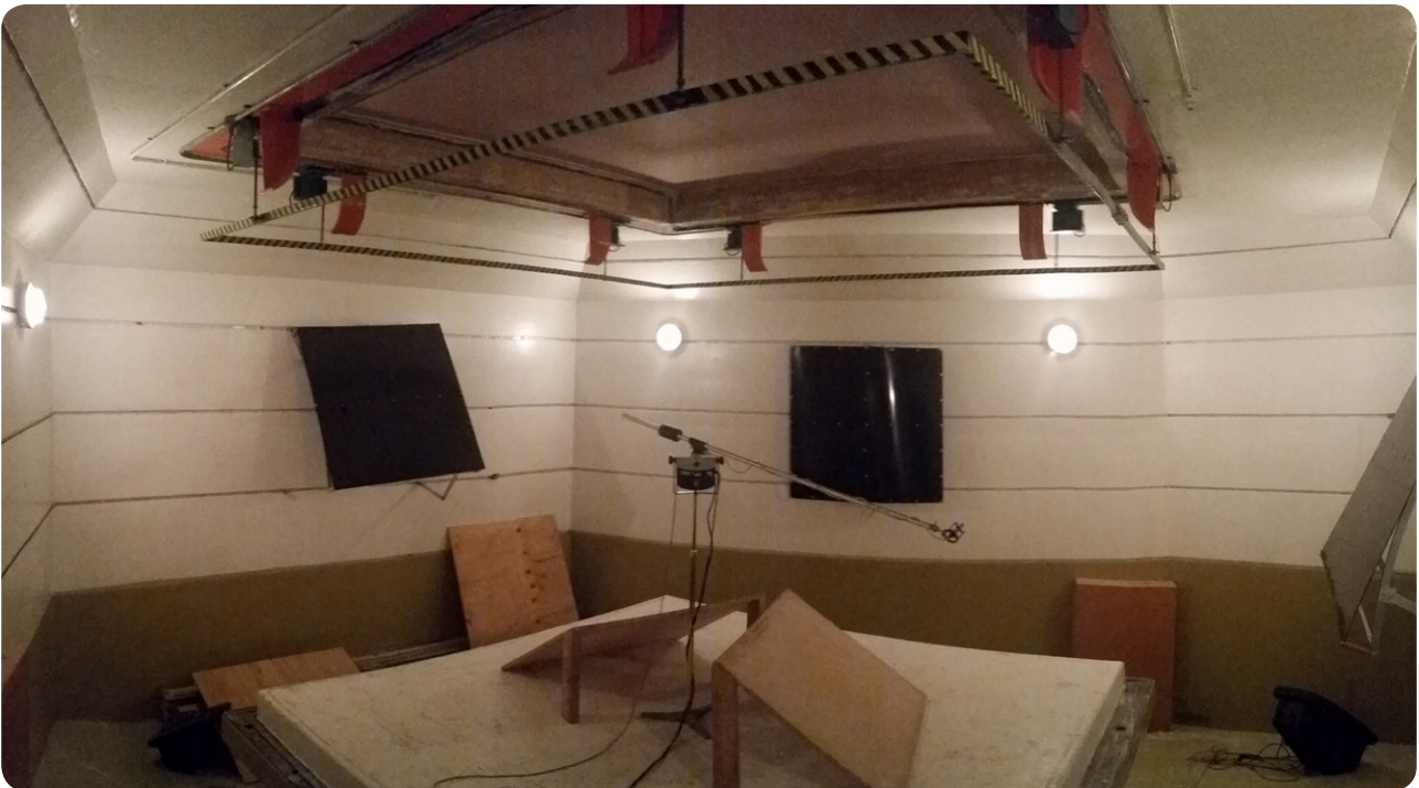
Figure 7.2: Reverberation Chamber B with CLT floor and direct fixed plasterboard installed.
