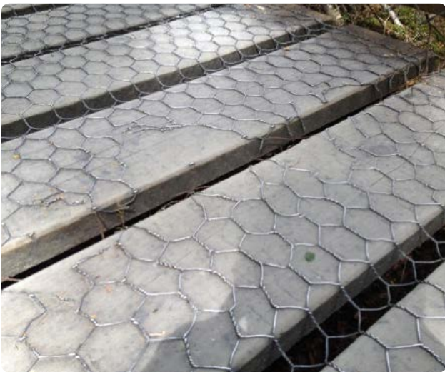
Figure 3.43: Wire netting attachments.
