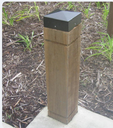
B: Flush-faced – Rebating bollard ends allows caps to fit flush with column sides, giving a more complex but neater finish.
