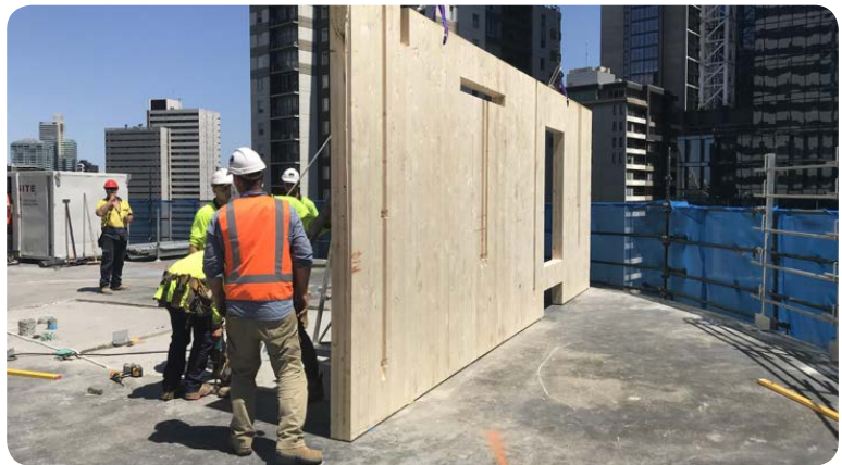
Figure 7.1: A 10-storey vertical extension to an existing six-storey office, this Melbourne hotel designed by BatesSmart for Hume Partners Property would not have been possible without timber. With the existing office building only capable of accommodating an extra six storeys in concrete, the project team turned to a CLT and Glulam solution, finding the lighter weight system allowed an extra four storeys for a total height of 16 storeys. Images: http://atelierprojects.com.au/
