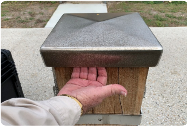
Figure 5.10: Finger entrapment.
