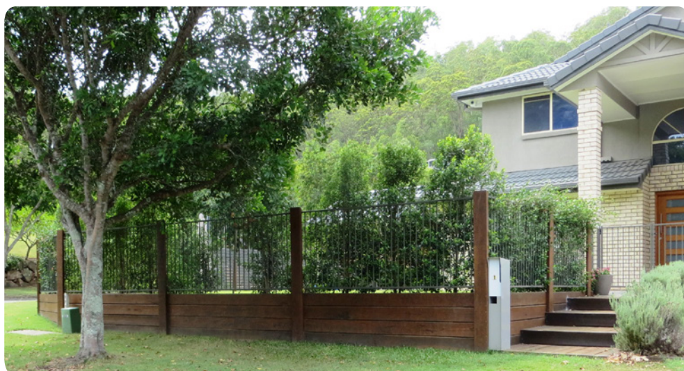
Figure 4.2: Hardwood retaining wall and fence posts being maintained with CN oil.
