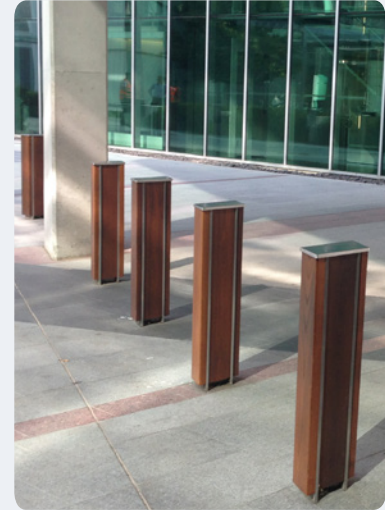
C: Composite alternative – Fixing multiple smaller members in conjunction with stainless steel fins and capping provides a sophisticated alternative to single mass timber elements. Those pictured provide crash protection at an airport.
