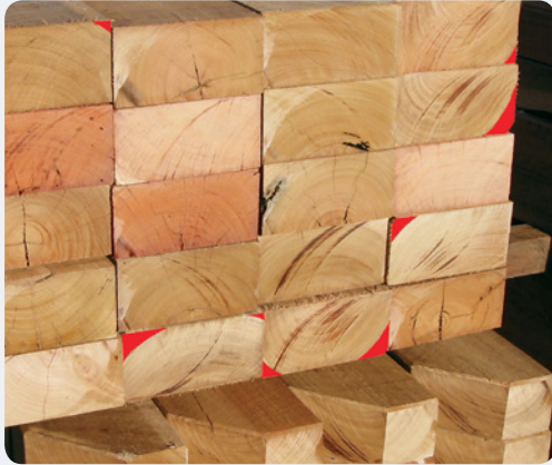
A: Extent of treatable sapwood in hardwood. Picture shows sapwood (highlighted in red) in untreated hardwood bollards. It is not possible to speak in a meaningful way of treating hardwood sapwood beyond H3.
