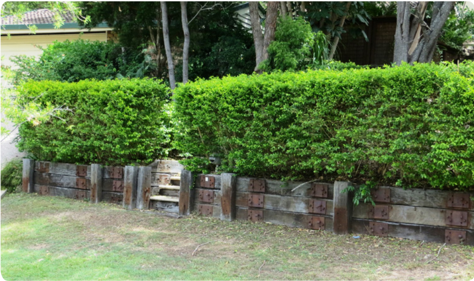
Figure 2.3: Recycled hardwood railway sleepers complete with rail bearing plates.
