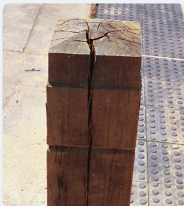
A: Uncontrolled splitting – Bollards that contain heart (pith) frequently split along their length.
