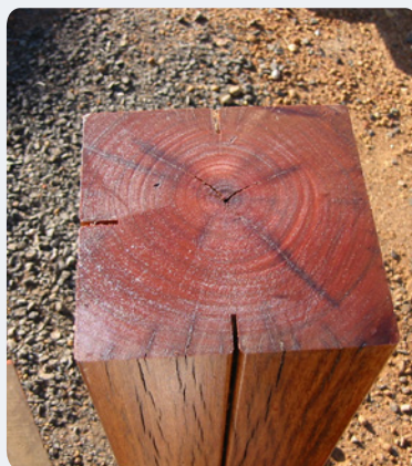
B: Controlled movement – Using a router to provide a groove over a saw line controls surface splitting and avoid splinters.
