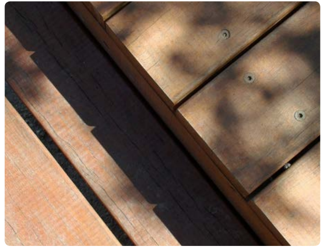
Figure 3.20: Incorrect orientation of boards at landing.
