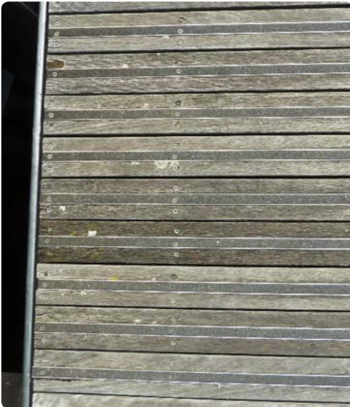
Figure 3.29: Boards with inlaid grit straps.
