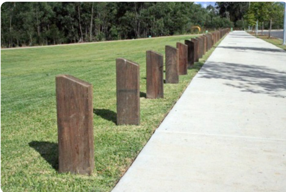
Figure 2.1: Parks frequently use timber bollards to guide pedestrians and define borders. Photograph: Dennis Clark Photography
