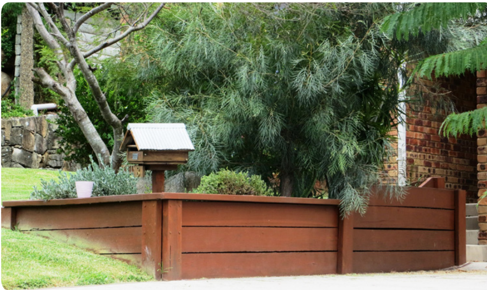
Figure 2.2: High quality hardwood sleepers
