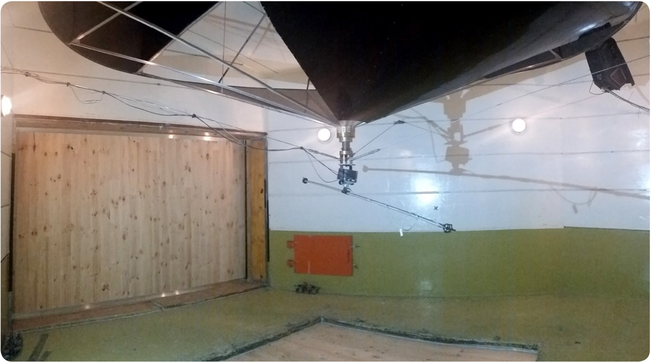
Figure 7.1: Reverberation Chamber A with bare CLT wall and floor installed.
