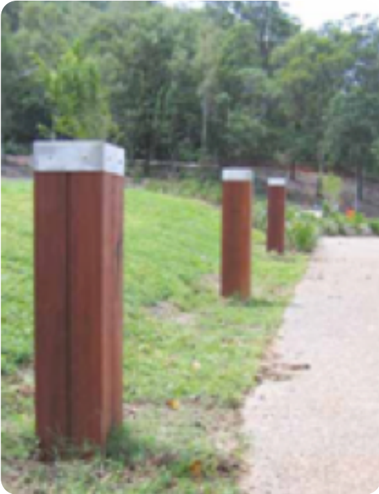
Figure 9.1: Timber durability is enhanced by applying appropriate paint and oil systems. The bollard shown is protected with a penetrating oil that repels water and blocks ultra-violet radiation.
