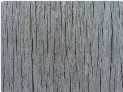
Figure 3.5: Naturally textured surface from weathering.
