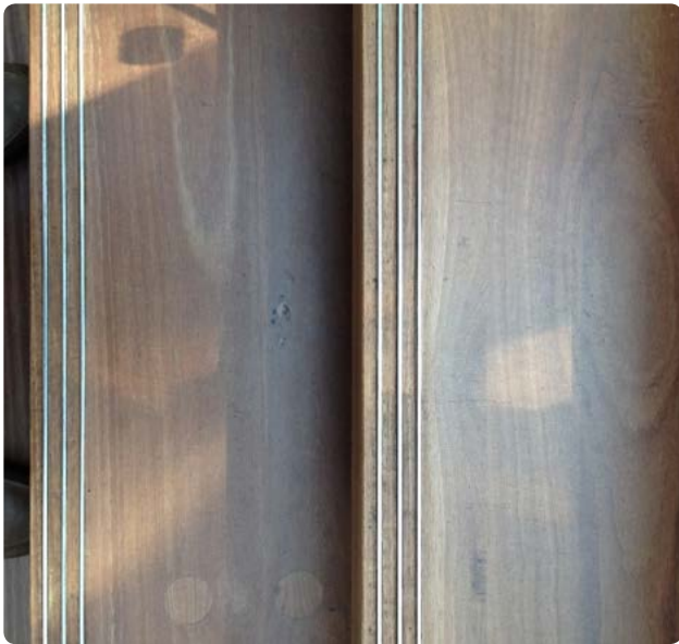
Figure 3.32: Metal ribs at stair tread nosings.
