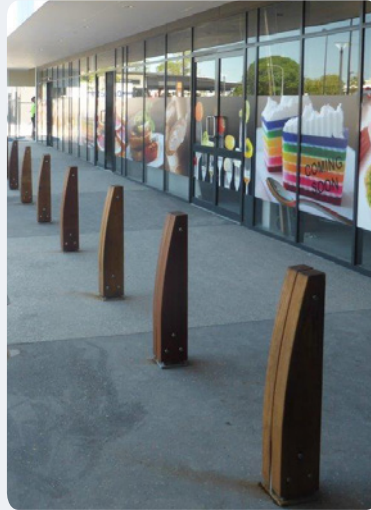
B: Composite alternative – Two wide members are fixed to a central steel fin, providing a mass appearance.
