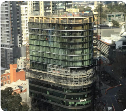
Figure 7.1: A 10-storey vertical extension to an existing six-storey office, this Melbourne hotel designed by BatesSmart for Hume Partners Property would not have been possible without timber. With the existing office building only capable of accommodating an extra six storeys in concrete, the project team turned to a CLT and Glulam solution, finding the lighter weight system allowed an extra four storeys for a total height of 16 storeys. Images: http://atelierprojects.com.au/
