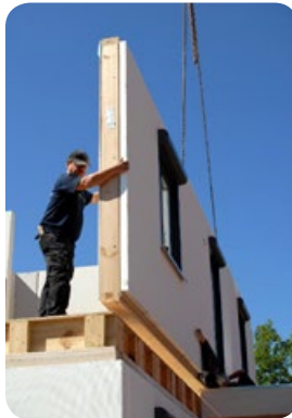
Figure 6: Prefabrication-intensive construction – panel construction.
