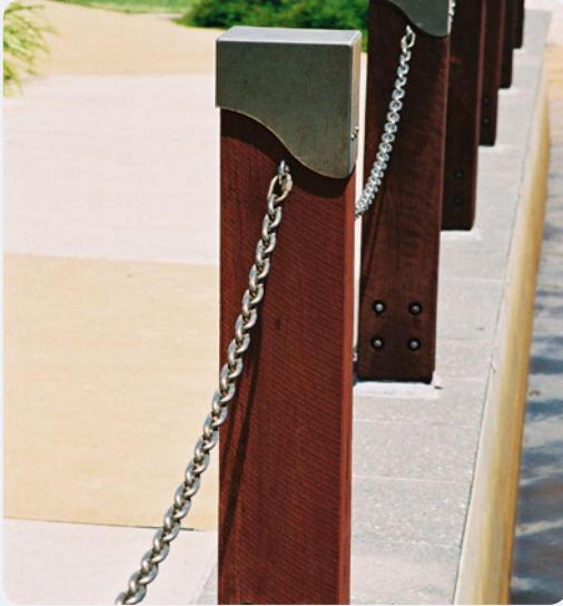
A: Rope and chain – Linking bollards restricts vehicle movement and discourages pedestrian access with minimal visual intrusion. Copyright Dennis Clark Photography
