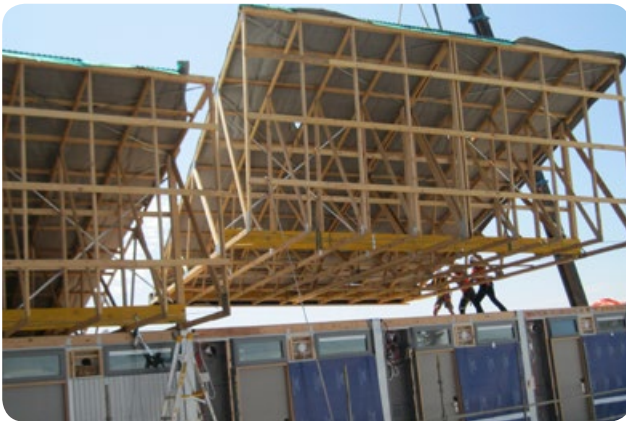
Figure 7: Site-based component assembly – roof modules
