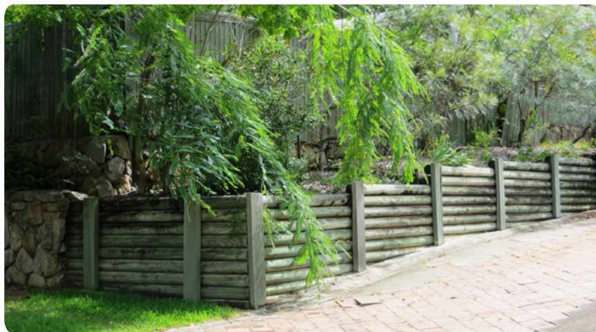
Figure 2.1: Combination of durable hardwood posts and H4 CCA treated rounds
