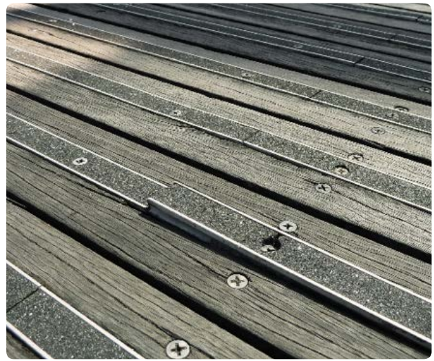
Figure 3.42: Dislodgement of inset straps.
