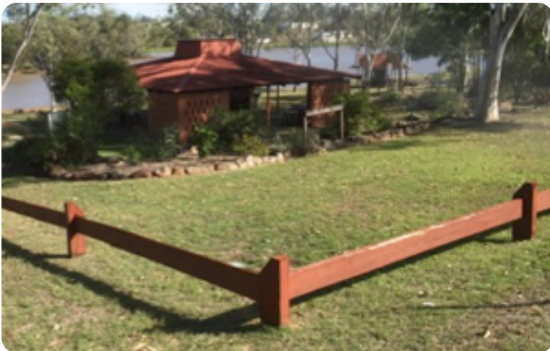
Figure 10.1: Original timber barriers at Lake Apex, Gatton, Queensland. The exposed hardwood shows some weathering but is still functioning after 30 years exposure, some areas experienced extended areas of submersion.
